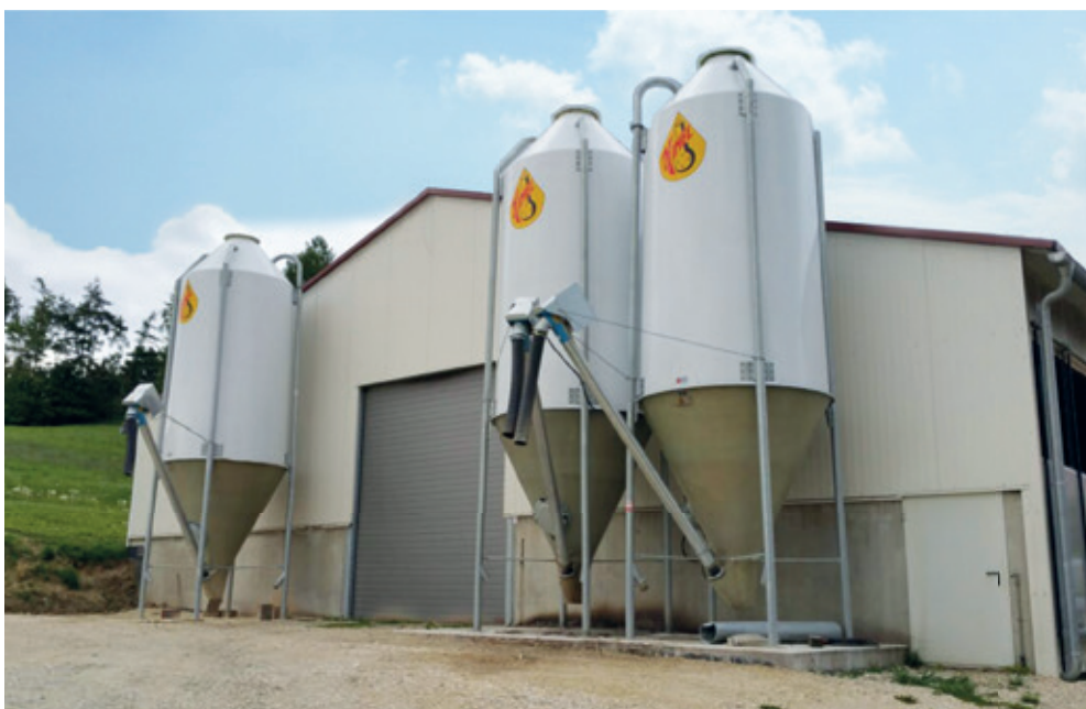
HIMEL GRP mixed feed silos with augers
