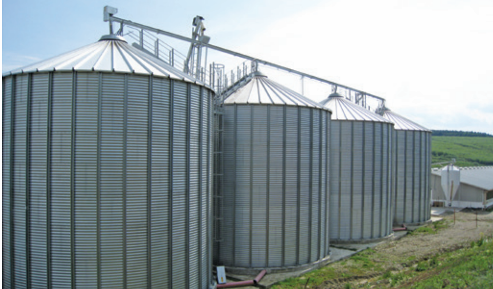
HIMEL outdoor silos with filling via trough augers
